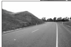
Left: the new curve from the north. Right: the finished product.
