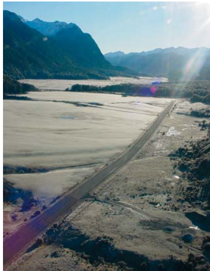
Milford Road - the only access to Milford Sound.
