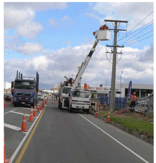
Below: Redundant power lines are removed.
